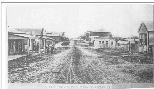
LOOKING DOWN MAIN ST OREPUKI
